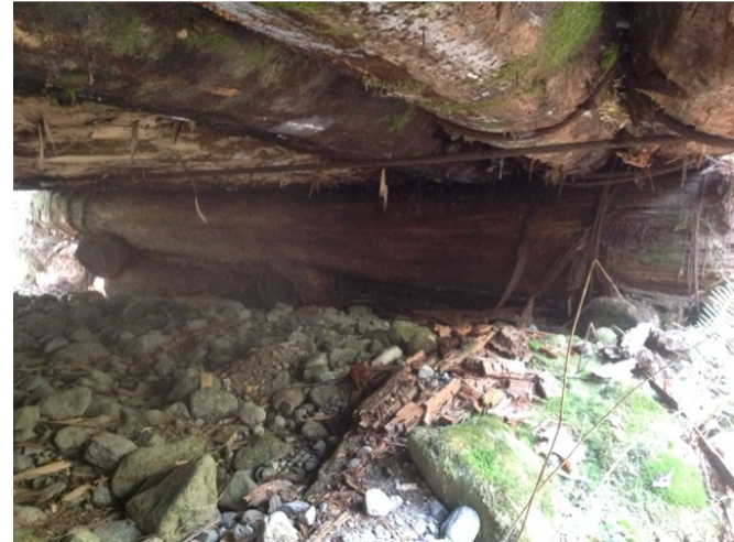
Right Bank Abutment when facing downstream
