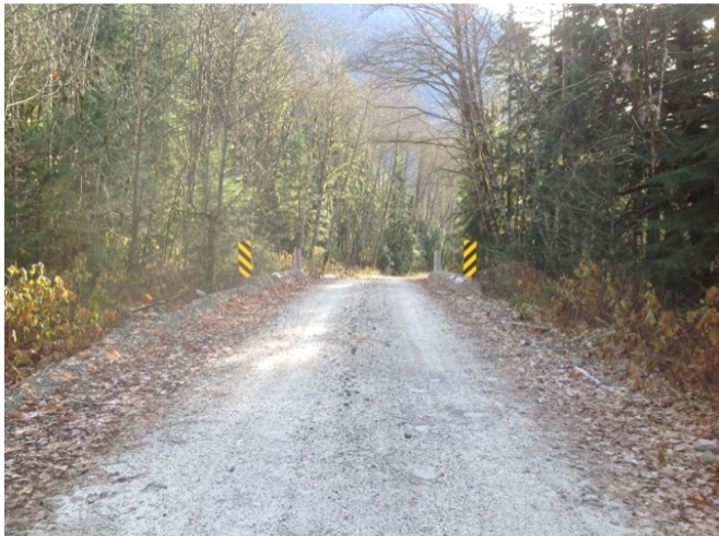
Approach from Right Bank when facing downstream
