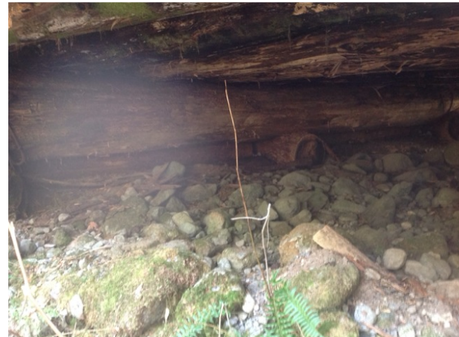
Left Bank Abutment when facing downstream
